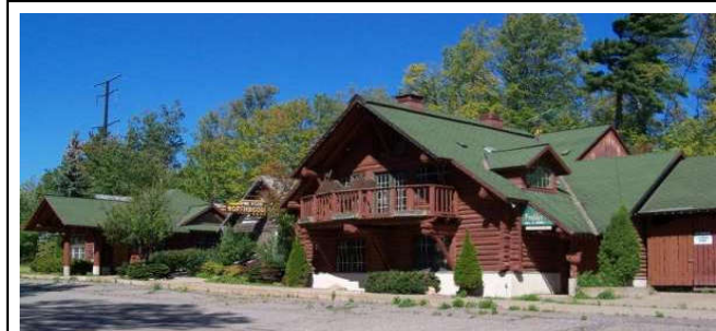
Project: 260 Northwoods, Marquette Township Grant funds budgeted: $6,300 Activities funded: revised Phase I, Brownfield plan
