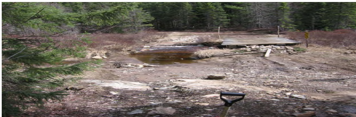
*Existing Mulligan Creek Crossing
