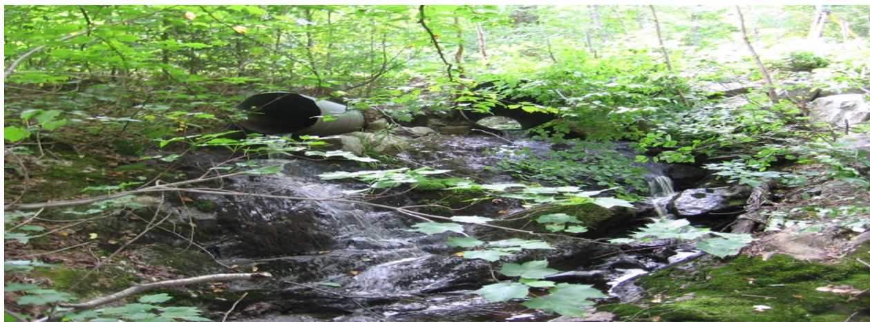
*Existing culvert at Trail 5 crossing of Mulligan Creek Tributary 1.
