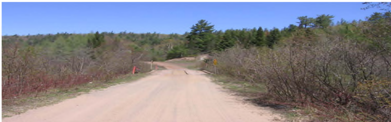
*Existing Dead River Bridge On Trail 5
